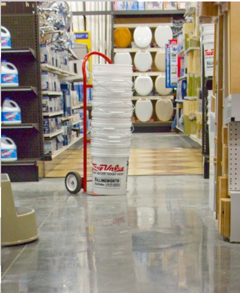
The exposed HardWear concrete floor in Killingworth True Value, Killingworth, CT, has a polish-like appearance and durability at much lower cost.
